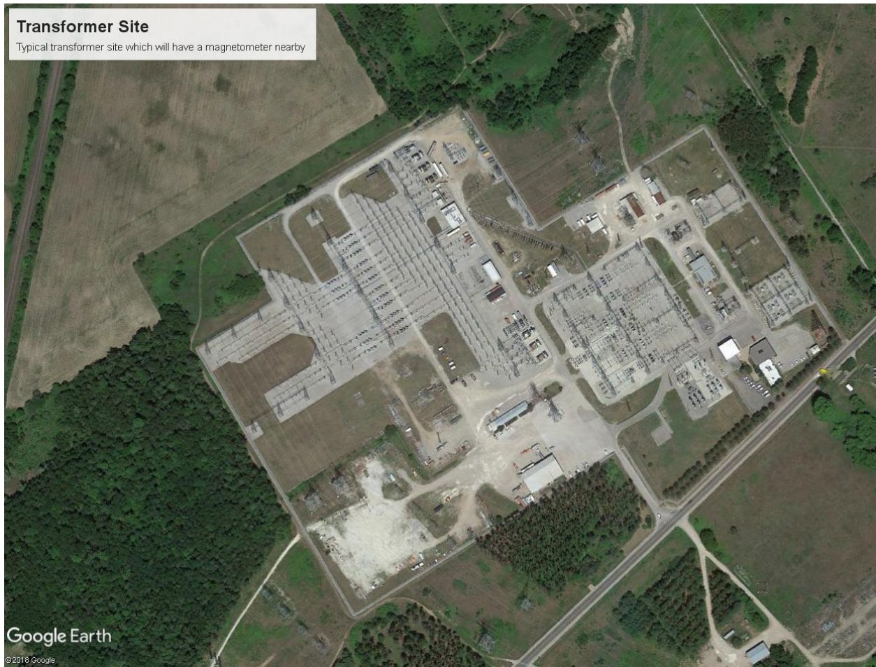
Fig. 5 Typical Ontario Hydro Transformer Site
