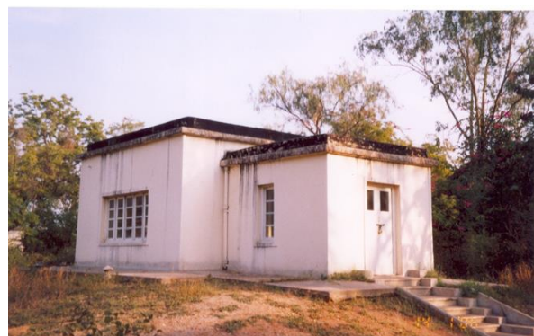
Fig. 2.1c: Secondary variometer building
