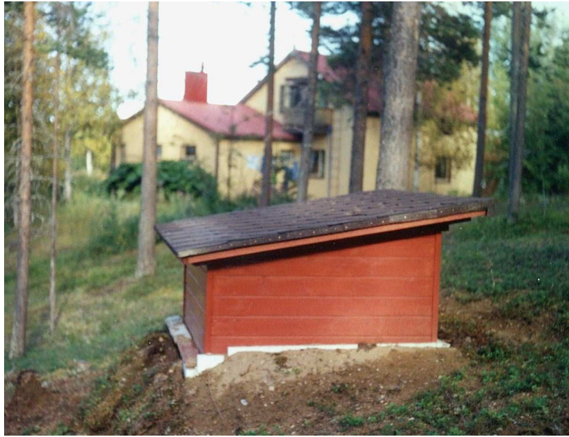
Figure 4: The magnetometer hut at the Pello (PEL) IMAGE station. The computer is in the house and data transfer is through optical wires.
